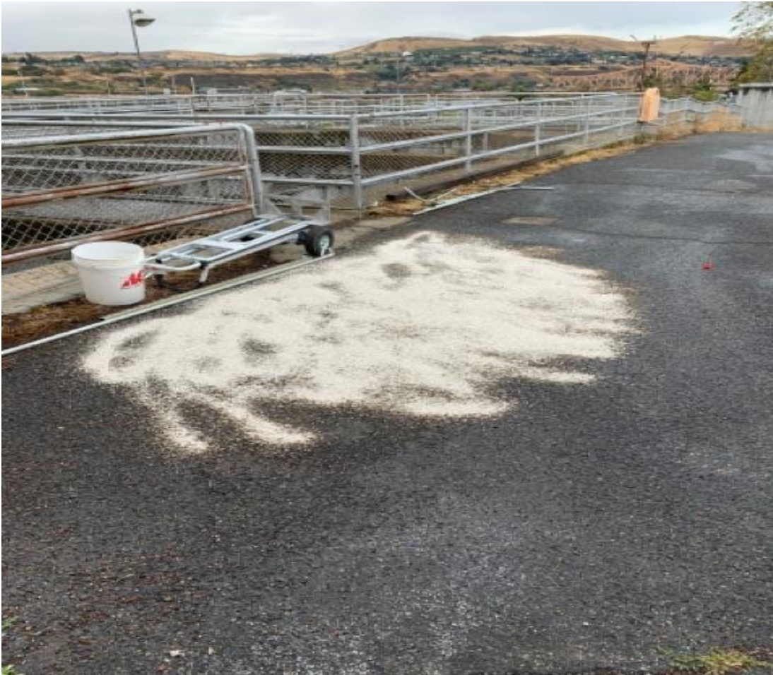
Small oil spill near north fishway exit. Absorbent containment. No oil made it to water
